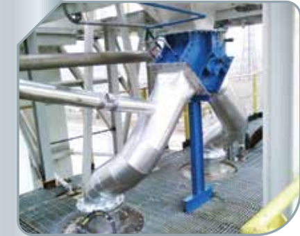
Pantolon klepe Flap type gravity diverter valve
