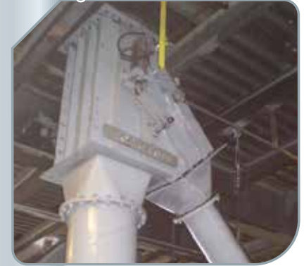
Pantolon klepe Flap type gravity diverter valve
